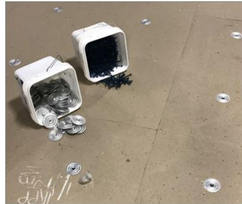
Parapet walls / flashing. Fasteners under roof membrane
